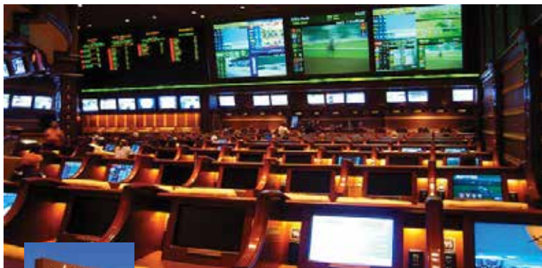
The Wynn Casino sends 66 sources to 125 displays. The system also includes 11 windowing processors, 14 audio endpoints, and SVSi's N-Command Controller.
